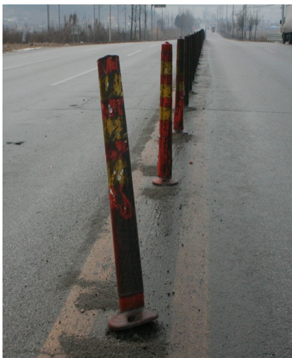
Damage due to insufficient fixing strength of the lower fixing plate
