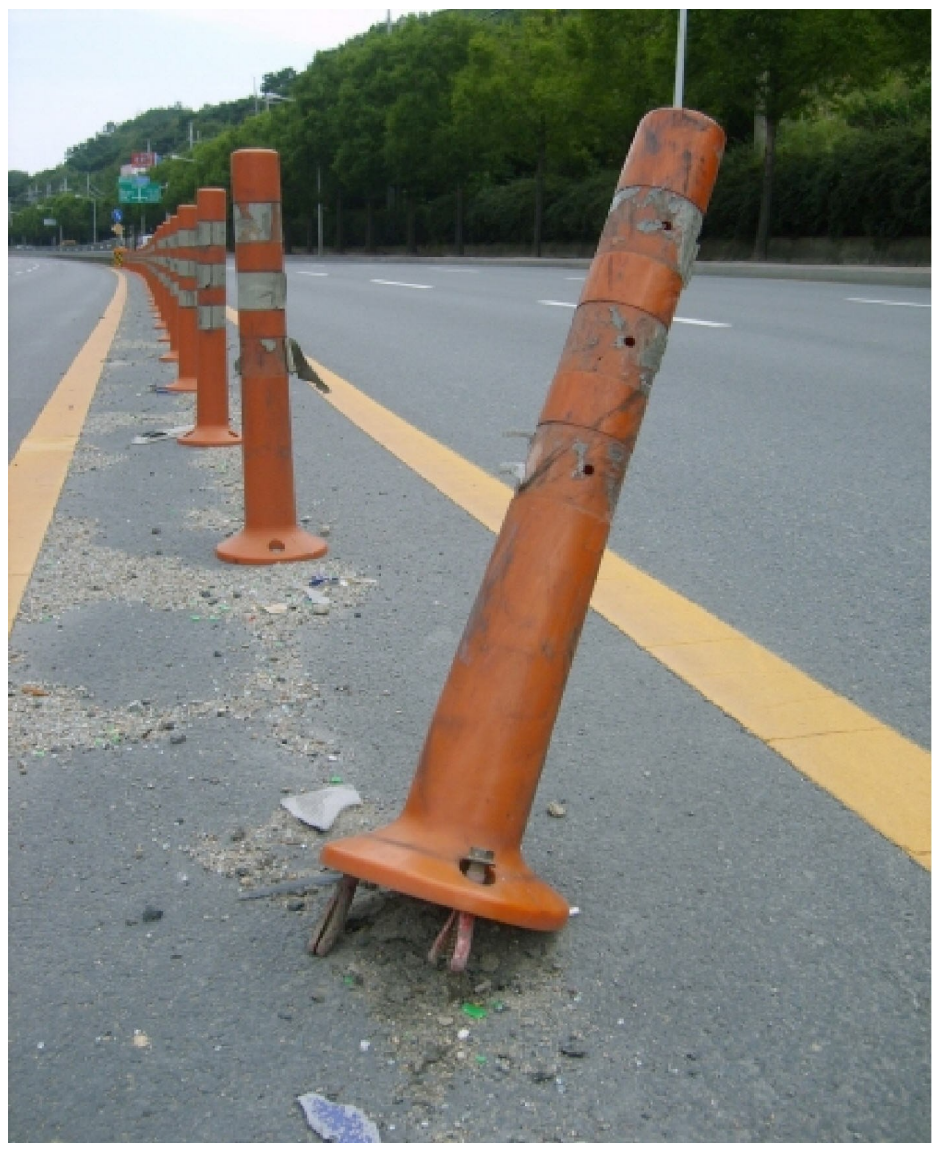
Damage due to insufficient bond strength
